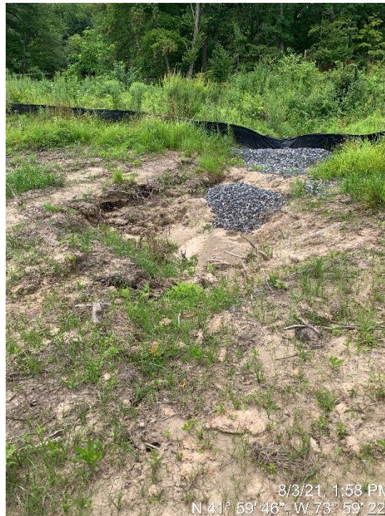
Photo 2: Silt fence in need of maintance
